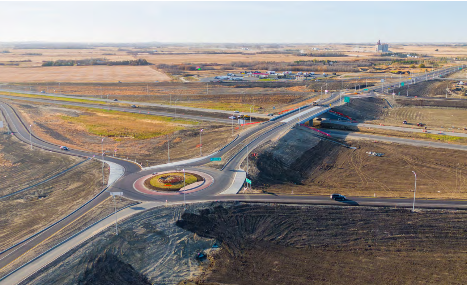
Regina Bypass Project, Parsons, Regina, SK
