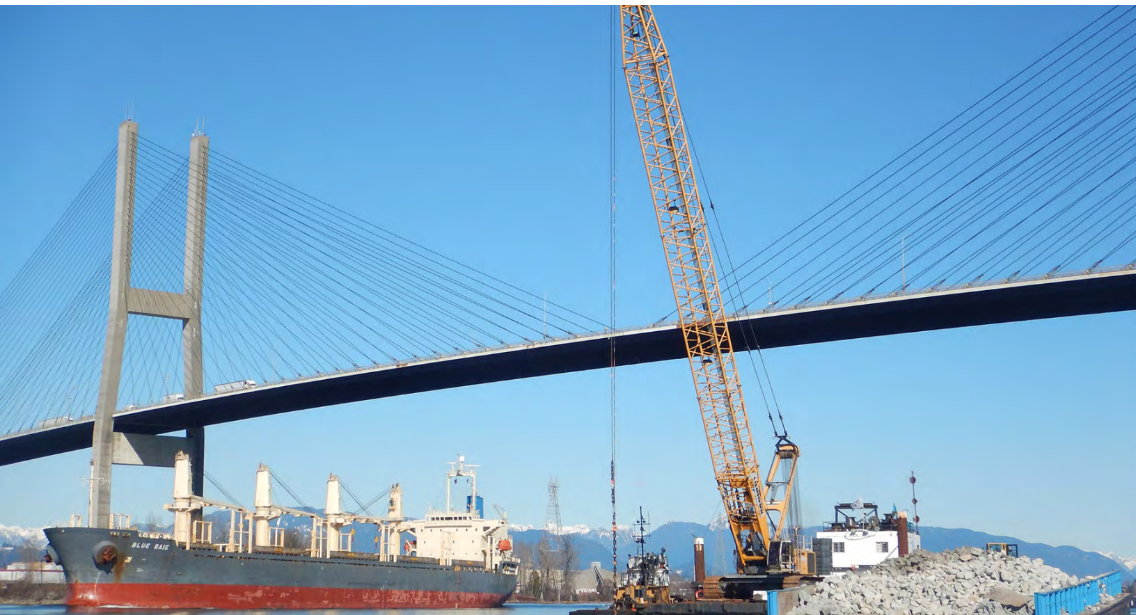
Scour Protection at the South Surrey Interceptor, Northwest Hydraulic Consultants Ltd., Fraser River, Delta, BC
