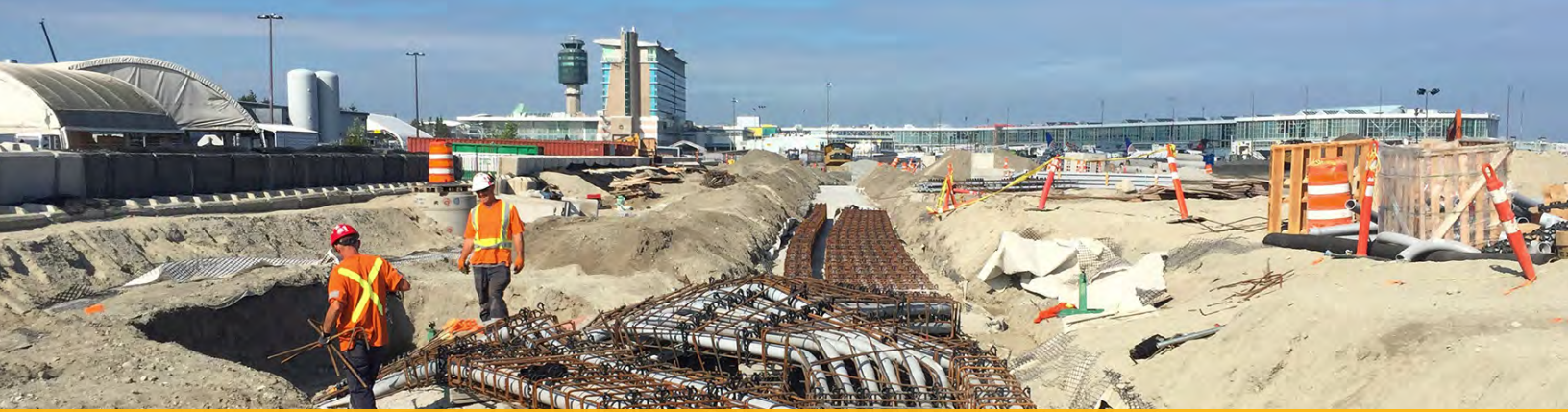
YVR East Apron VI Remote Stands, Hatch, Richmond, BC
