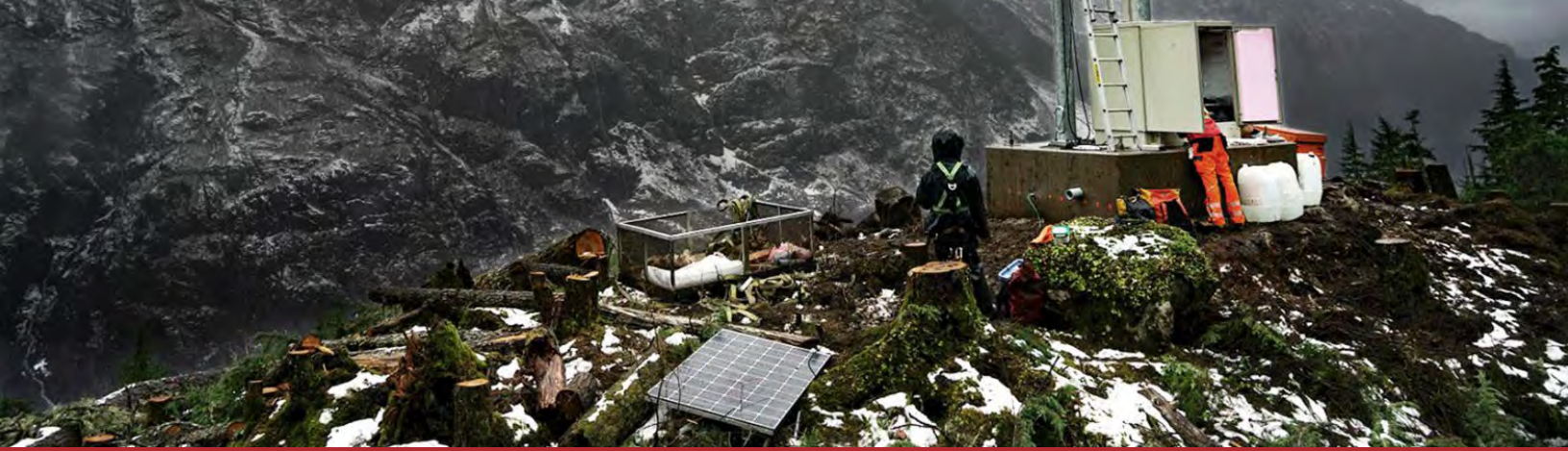
Automated Avalanche Detection System, PBX Engineering, Stewart, BC
