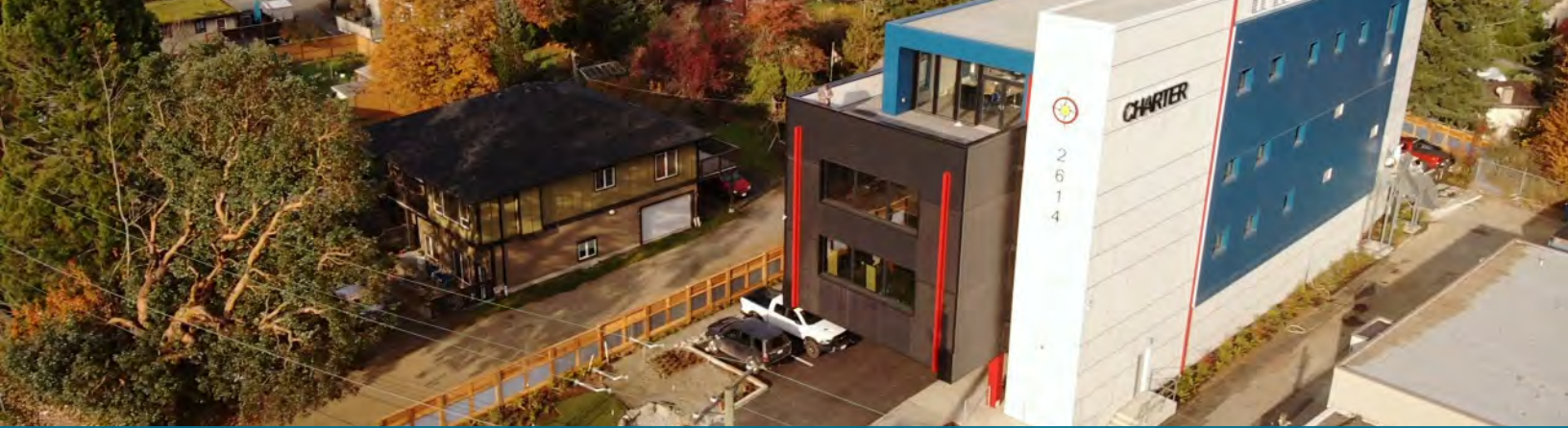
Charter Telecom Headquarters Passive Building, Morrison Hershfield Limited, Langford, BC
